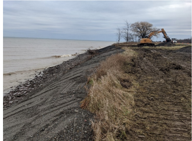
Placement of sediment from Johnson Creek along the LOSP bluff
